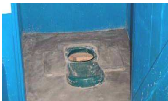
Fig. 5: Interior of a students' UDD toilet showing UD squatting pan (source: EcoSan Club, 2005)
