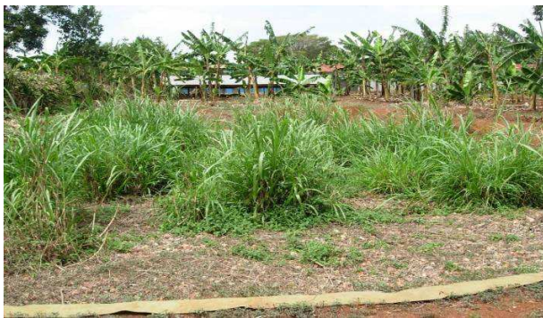
Fig. 11: Constructed wetland, planted with Elephant grass (source: EcoSan Club, 2005)
