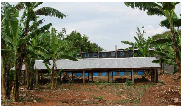
Fig. 12: Covered drying area for collected faeces from UDD toilets (source: EcoSan Club, 2005)
